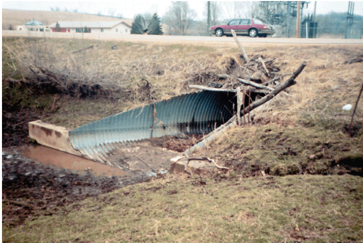
Figure 12 Metal Culvert
