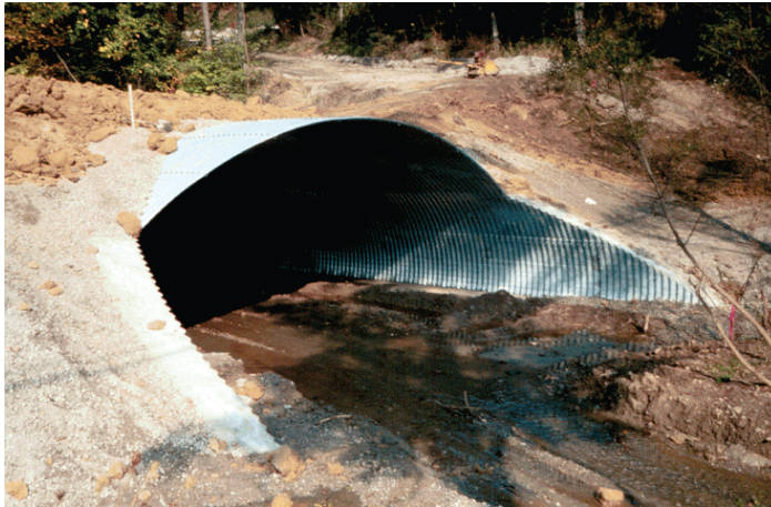
Figure 4 Pipe Arch Culvert
