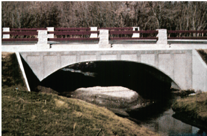
Figure 5 Arch Culvert
