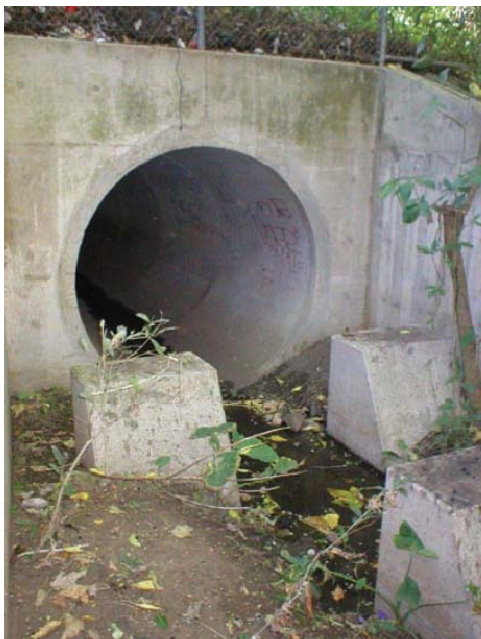
Figure 14 Energy Dissipaters
