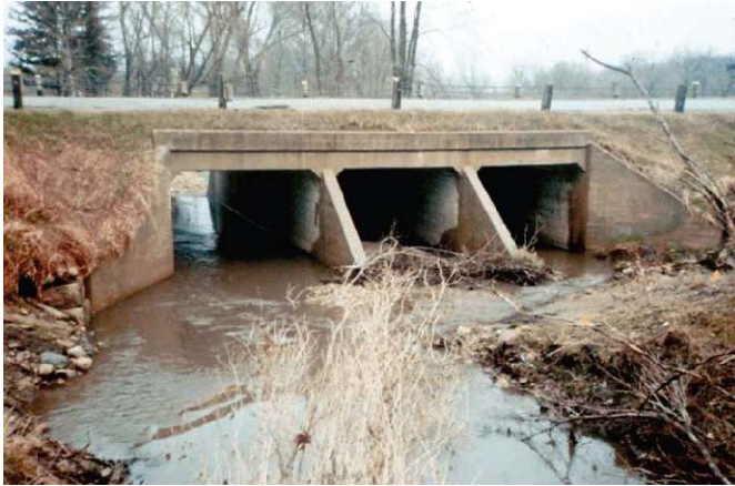
Figure 10 Frame Culvert
