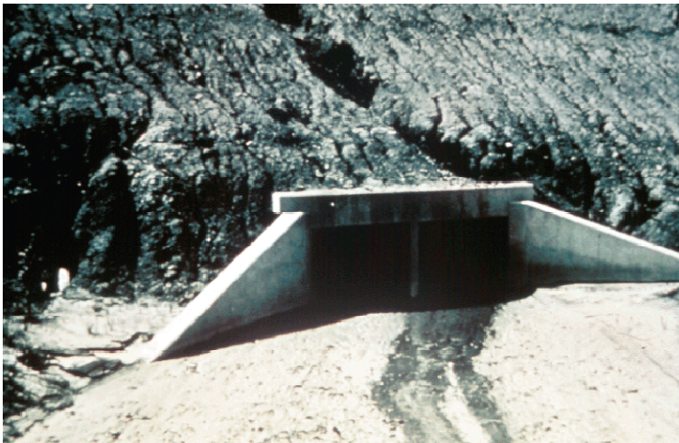
Figure 20 Scour and Undermining at Culvert Inlet
