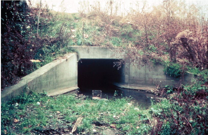
Figure 8 Concrete Box Culvert
