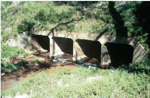
Figure. 9 Multiple Cell Concrete Culvert
