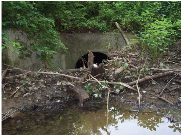
Figure 21 Debris and Sediment Buildup
