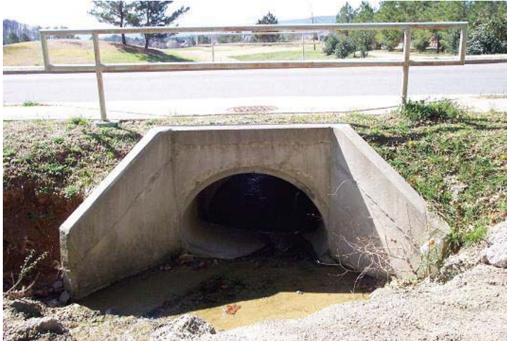
Figure 10 Culvert Mitered End
