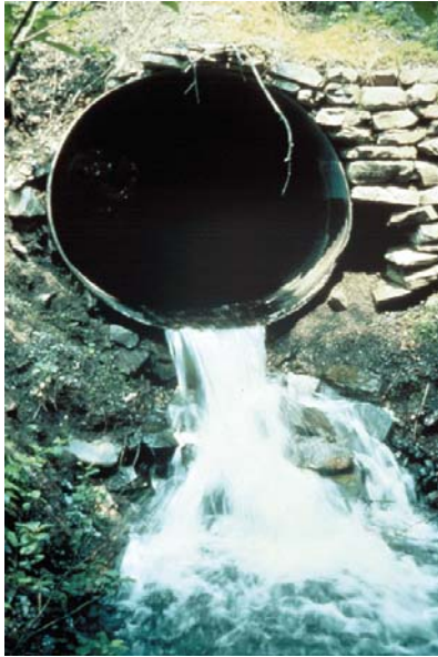
Figure ◦ Flexible Culvert
