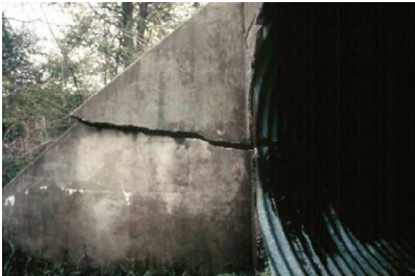
Figure 19 Cracking of Culvert End Treatment Due to Foundation Settlement
